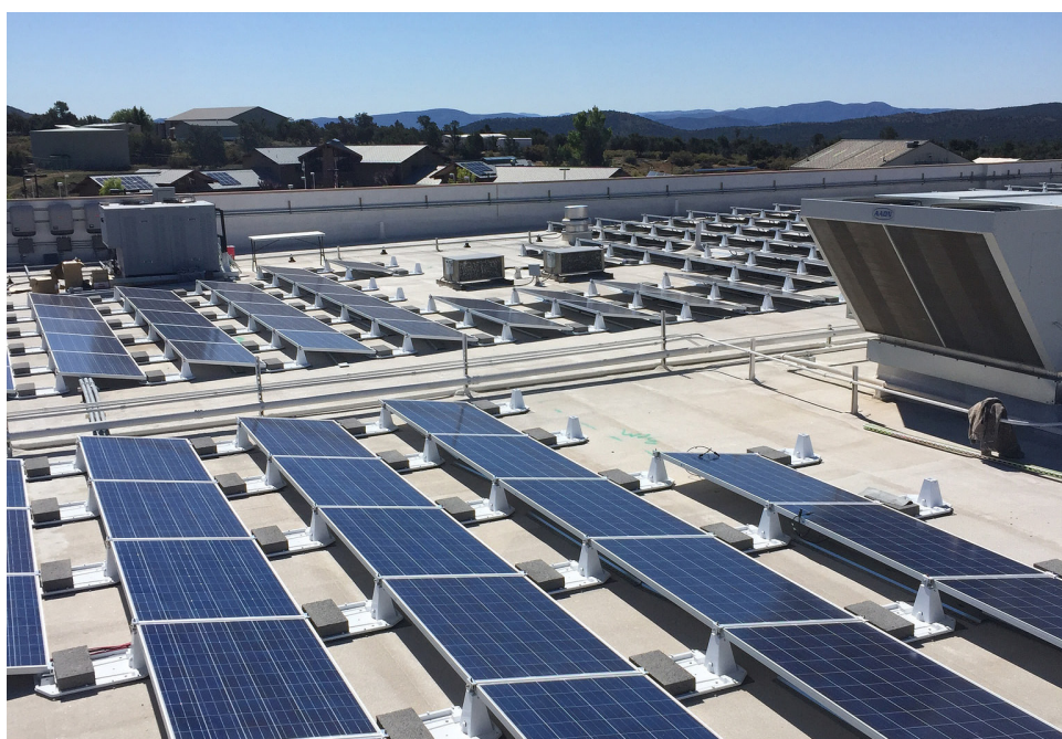
Solar array on ASU West Campus in Phoenix, Arizona
